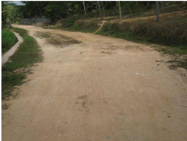
Fig. 2 Leveled subgrade before laying coir geotextiles
