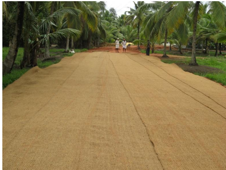
Fig. 2 Placing of coir geotextile - Mangalabharathy SN Kadavu road in Haripad
