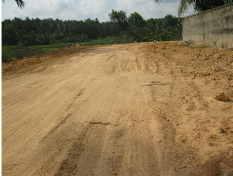
Fig.1 Before laying coir geotextiles Kozhinada
