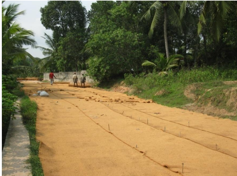
Fig. 3 Laying of coir geotextile in Kozhinada
