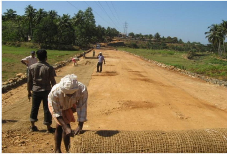
Fig. 1 Laying of coir geotextile in Chirakkad- Kumbakkad road (Varkala)
