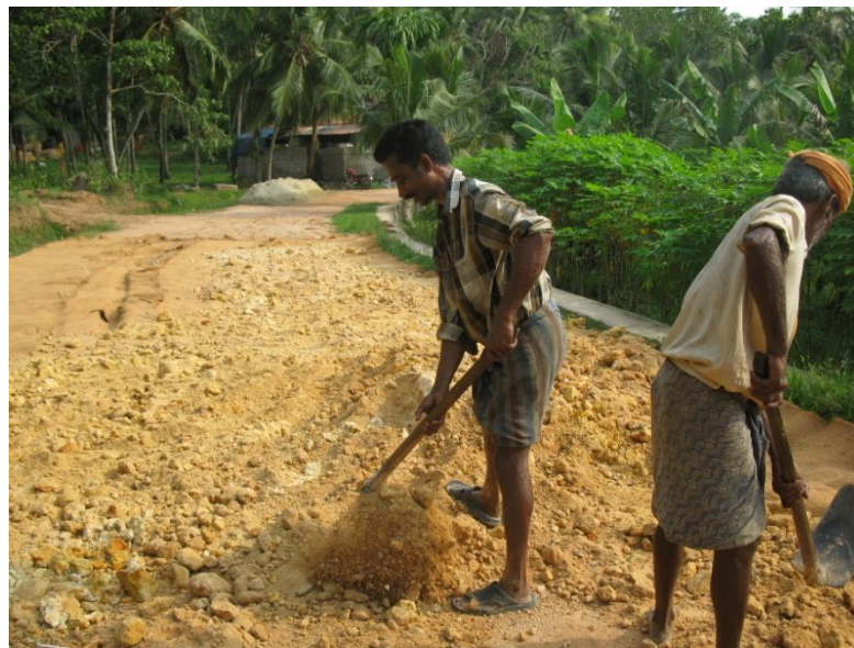
Fig. 4 Placing of soil above geotextile in Kozhinada
