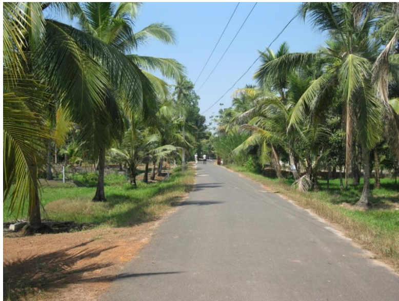
Fig. 4 Surfacing of road Mangalabharathy SN Kadavu road in Haripad
