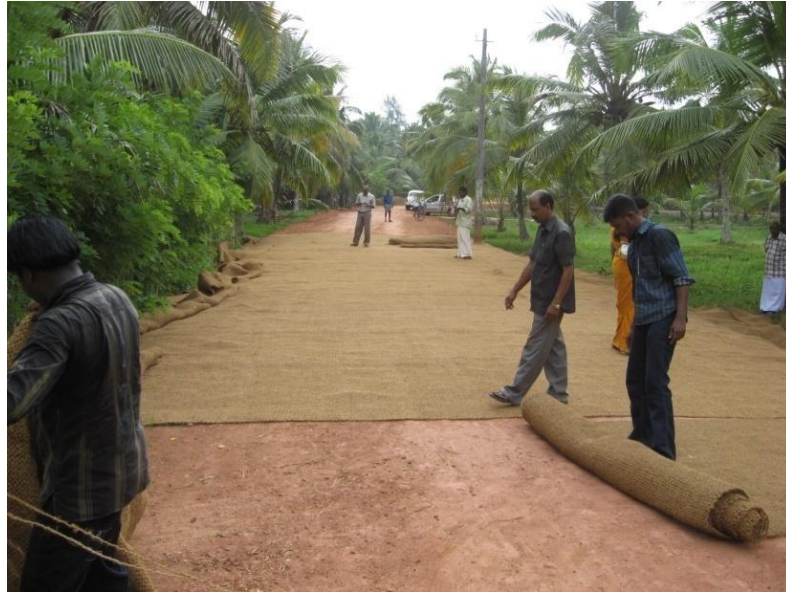
Fig. 1 Placing of coir geotextile – Mangalabharathy SN Kadavu road in Haripad
