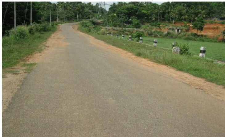
Fig. 3 Surfacing of road Chirakkad- Kumbakkad road (Varkala)
