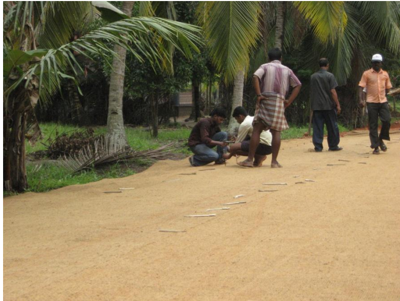
Fig. 3 Placing of coir geotextile Mangalabharathy SN Kadavu road in Haripad
