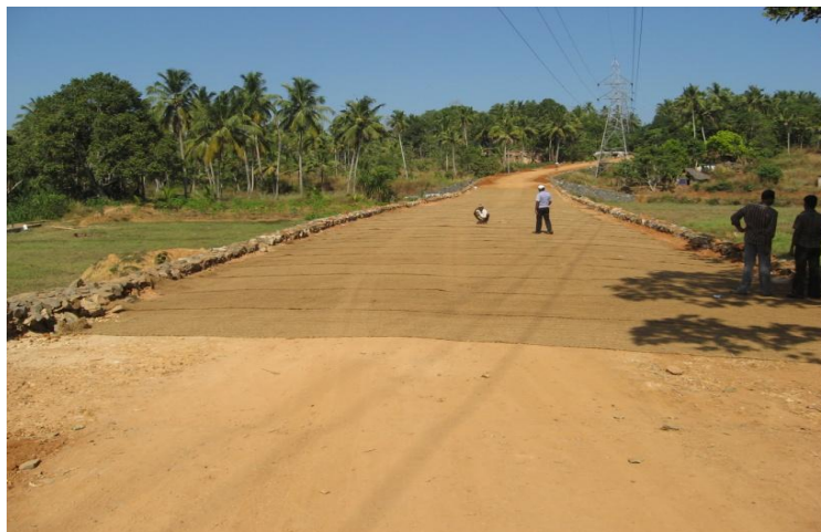
Fig. 2 Laying of coir geotextile Chirakkad- Kumbakkad road (Varkala)
