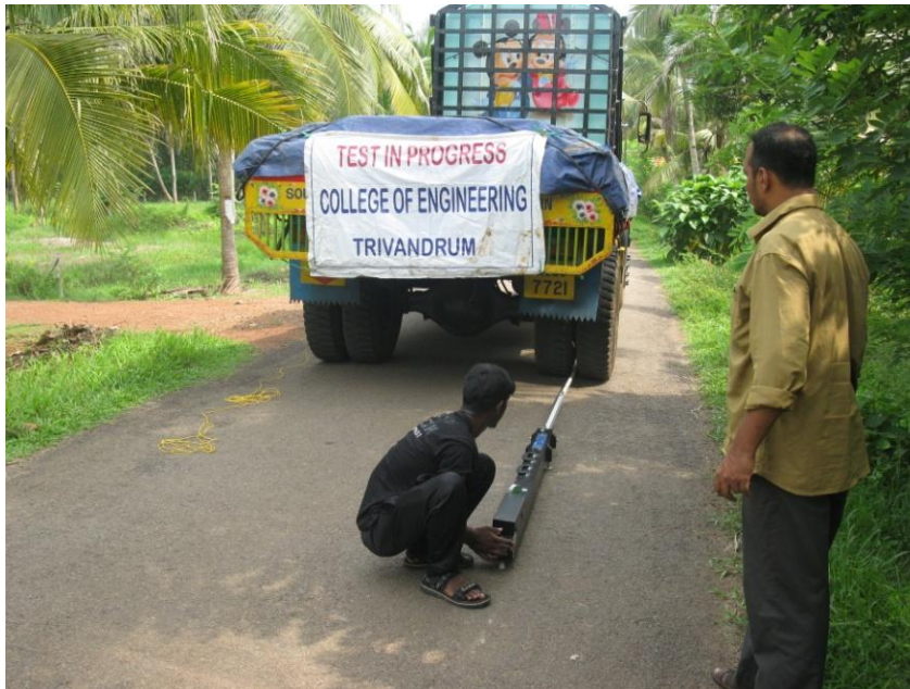
Benkelman Beam test in progress
